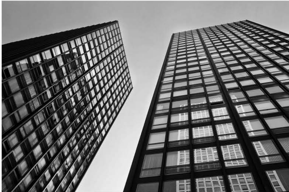
Mies van der Rohe 860-880 Lake Shore Drive Apartments. Photo by Assaf Evron 2014.
